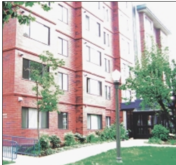
The E. B. Wilson apartment building had its venting system for boilers rerouted from sidewall to roof to eliminate exhaust fumes entering apartments making them unlivable.
