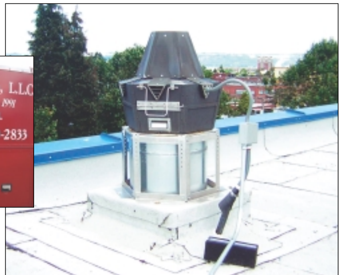
Above: Contractor Bill Crandell Right: Tjernlund VSAD AutoDraft® Inducer installed on roof of E. B. Wilson apartment building.
