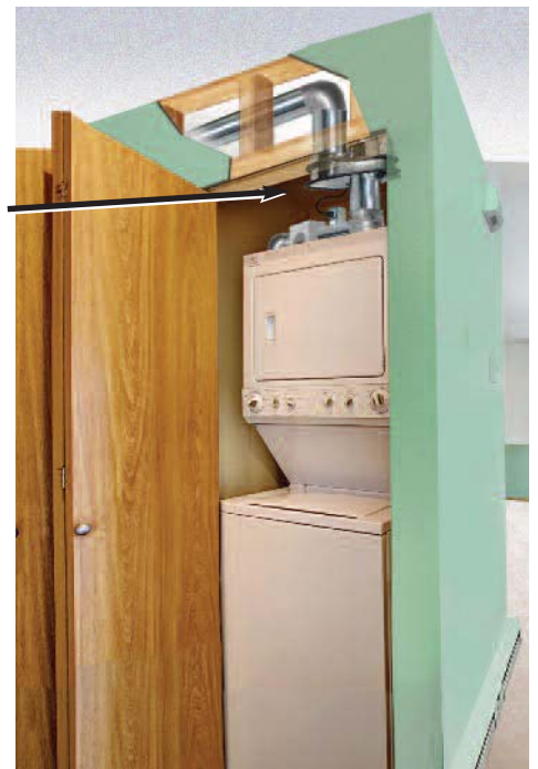
Typical Closet Installation
