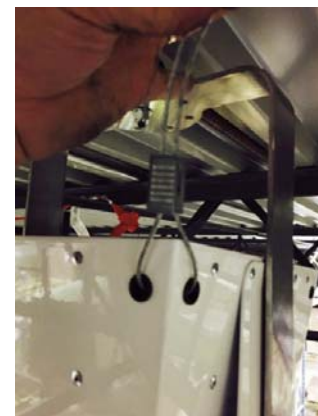
Feed cable back through clamp with minimum 6" tail.
