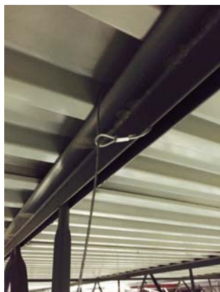
Loop safety cable around solid anchor point.
