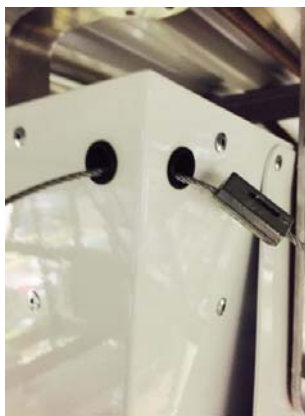
Feed cable with clamp through DSF2 holes.
