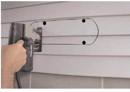
CUT OVAL TEMPLATE OPENING ALONG MARKED LINES.
